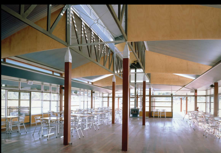
University of the Sunshine Coast Recreation Building - natural ventilation and lighting
