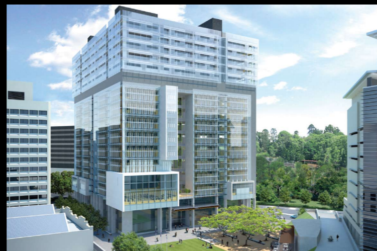
Brisbane Supreme Court and District Courts - under construction
