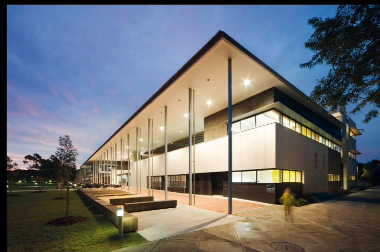
University of the Sunshine Coast Chancellery - mixed mode ventilation systems / reverse masonry veneer construction
